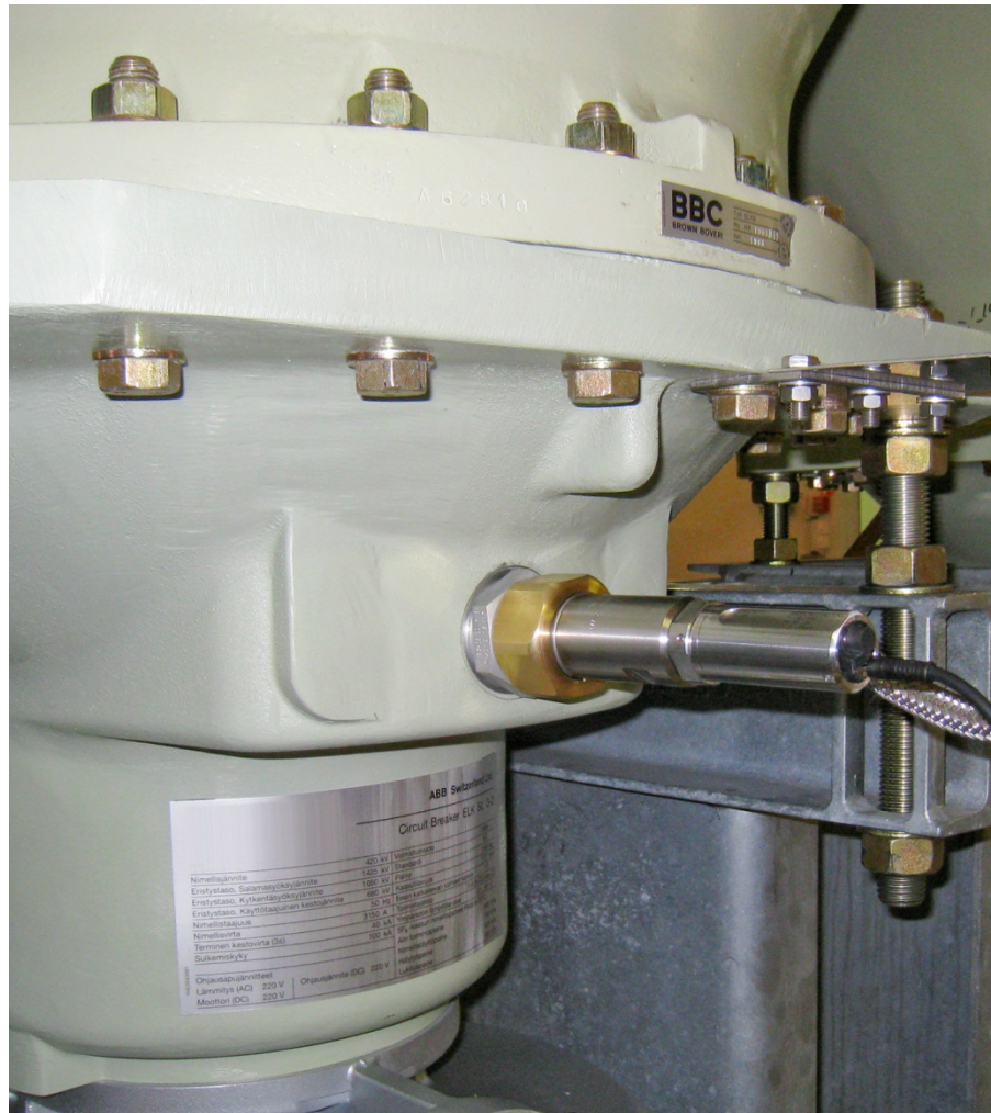
Figure 7 Indoor Installation in a Circuit Breaker
